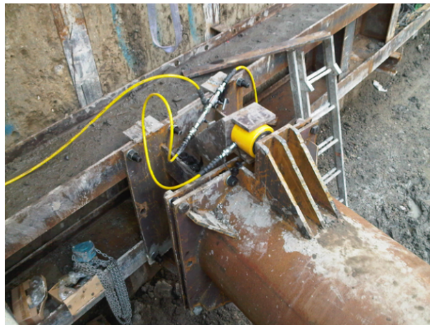
Picture of the post tensioning system
