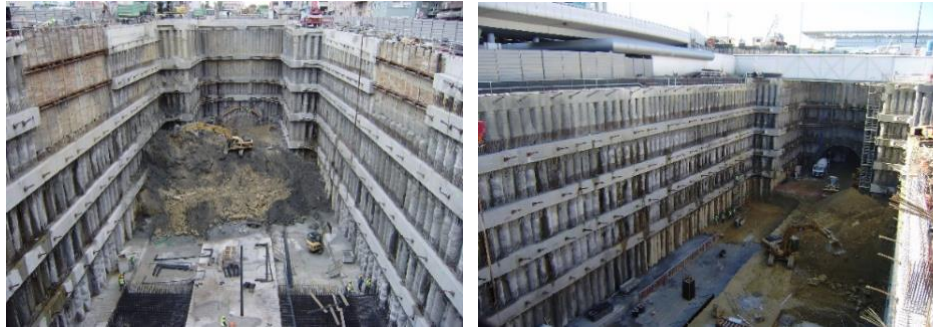
View of the excavation sites (Moscavide and Airport)
