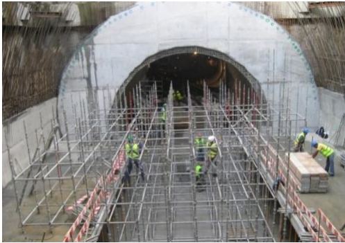
Execution of cut and cover galleries
