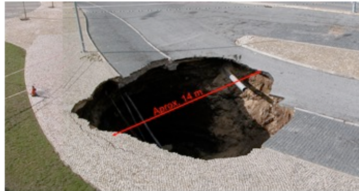
Post collapse images illustrating its consequences on the road pavement causing a bus to fall into the formed crater
