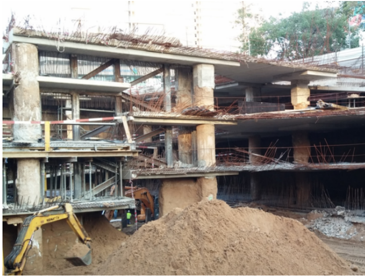
Partial view of the site during the excavation phase
