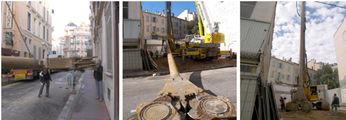
Installation of the equipment
