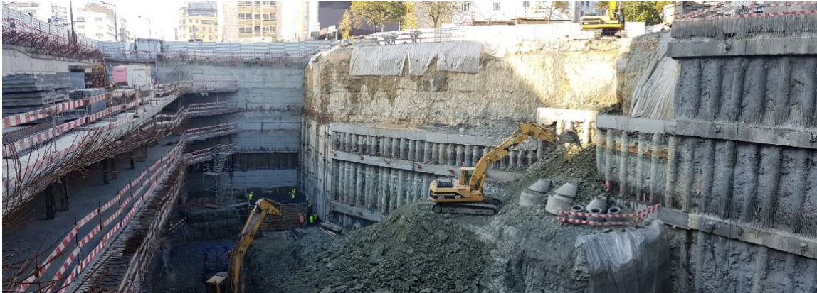
View of the final excavation works
