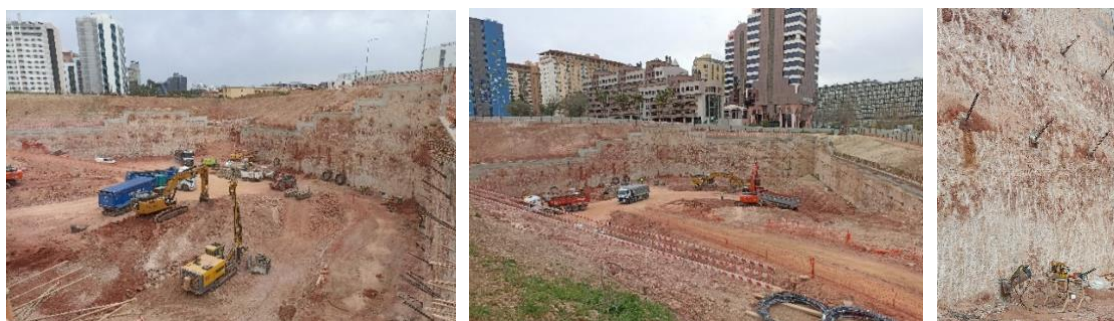
Excavation works and temporary ground anchors
