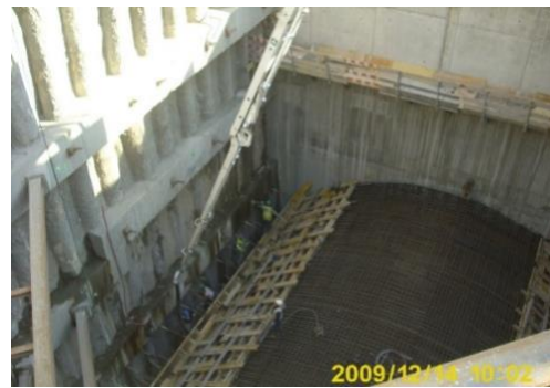
Execution of cut and cover galleries
