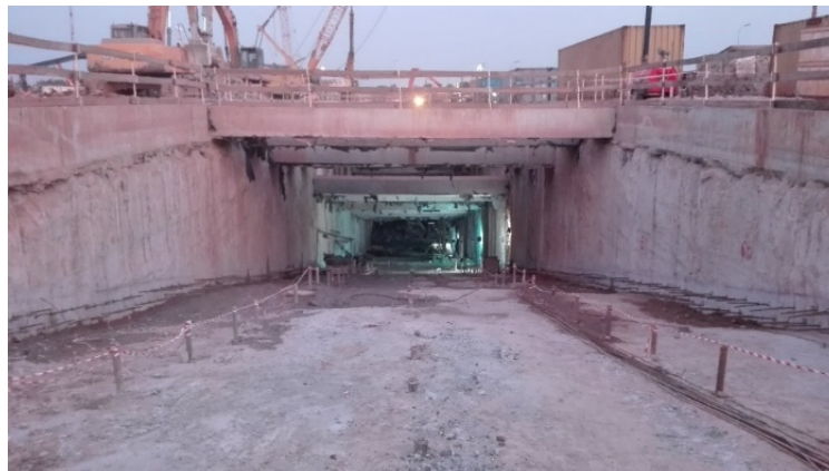
Trench in the execution phase of micro piles
