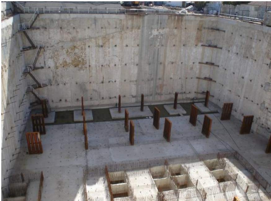
Conclusion of the raft foundation slab enlightening the injection pipe location
