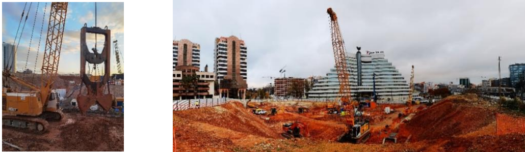
Excavation preliminary works and execution of diaphragm walls
