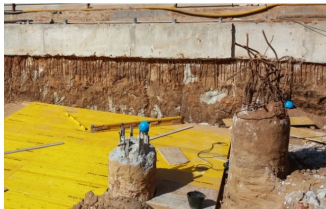
Picture of the beginning of the execution of the roof slab
