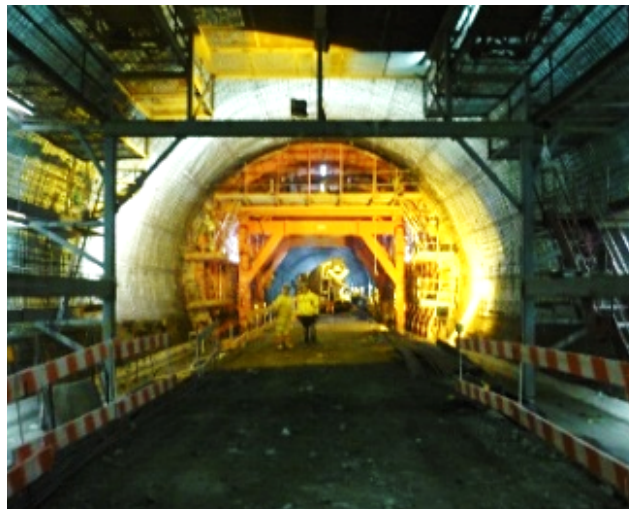
Installation of the waterproofing system and lining reinforcement
