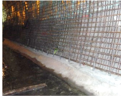
Detail of the side-wall-footing connection of the final lining
