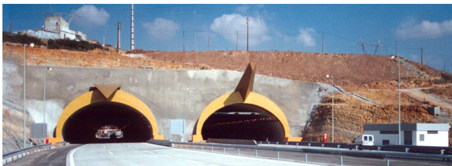
Overview of the Western Portal
