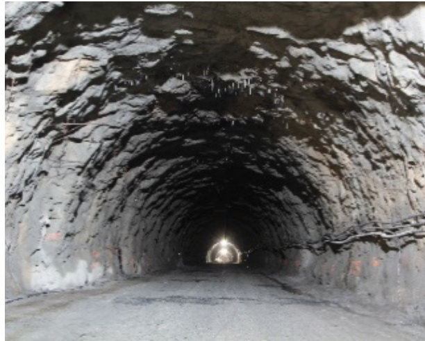
View of the excavation section
