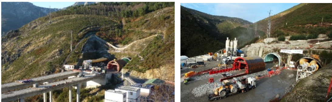
View of the east and west tunnel portals
