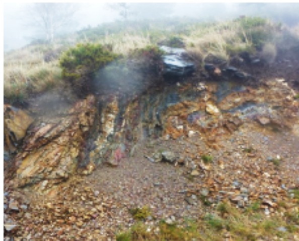
View of a fault zone on a road slope, at PK16+000
