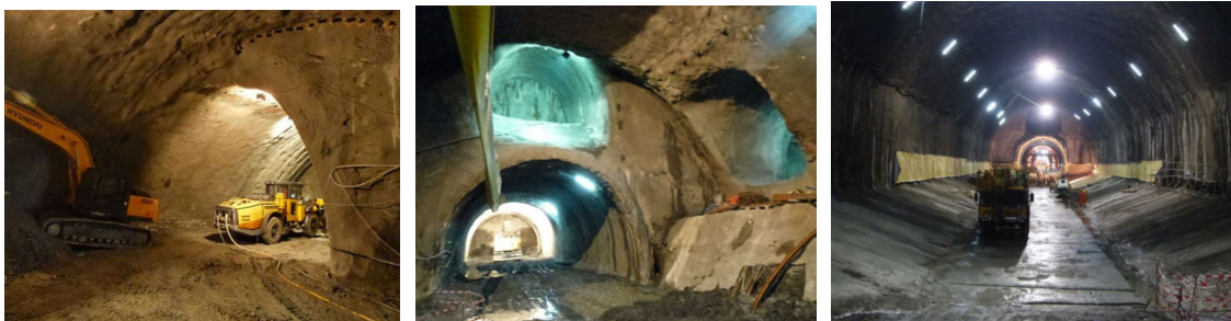
Pilot tunnel and final section of the Ali Boumendjel Station
