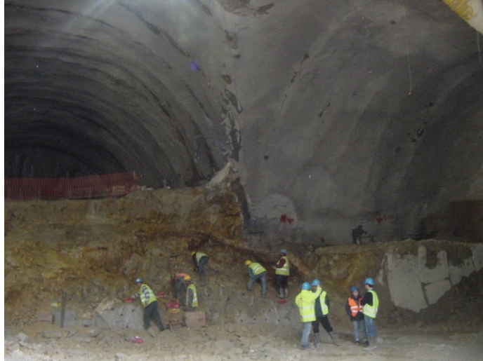
Intersection between main gallery and transversal gallery
