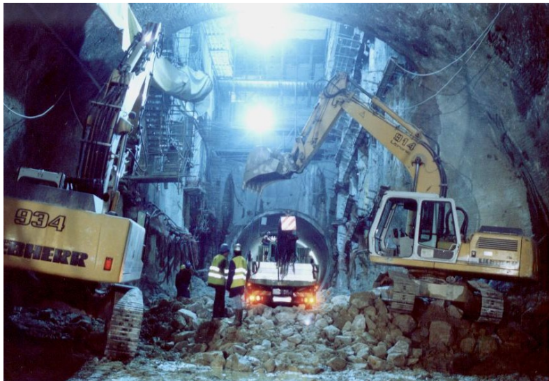
Excavation from the shaft at Fernandes Tomas Street
