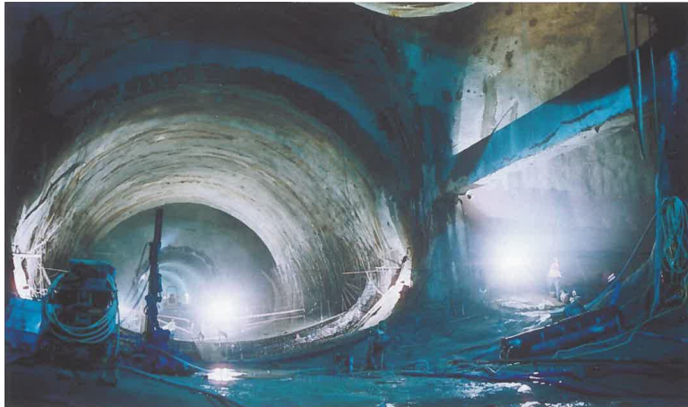
General view of the intersection area after completion of excavation
