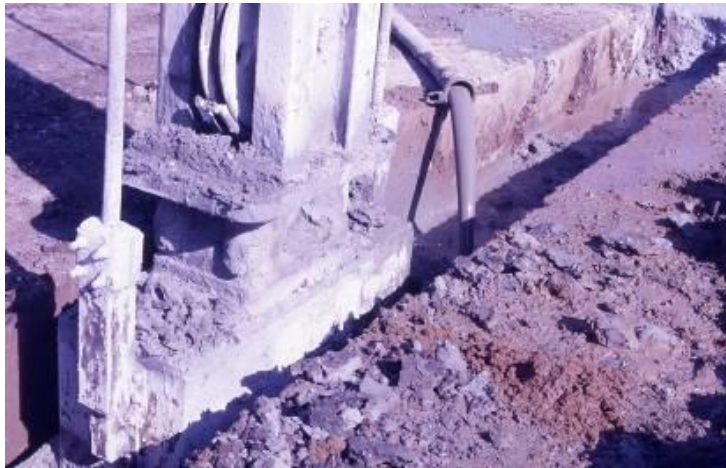
Corumana dam - Detail of diaphragm wall construction
