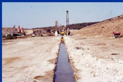
Flexible diaphragm wall
