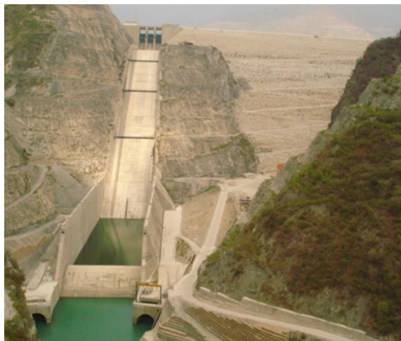
Theri dam - downstream view of the spillway
