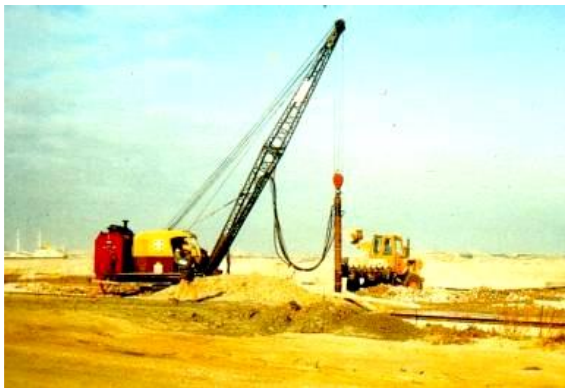
Equipment and methodology for vibroflotation
