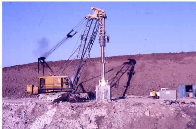
Corumana dam- equipment for the construction of the diaphragm wall
