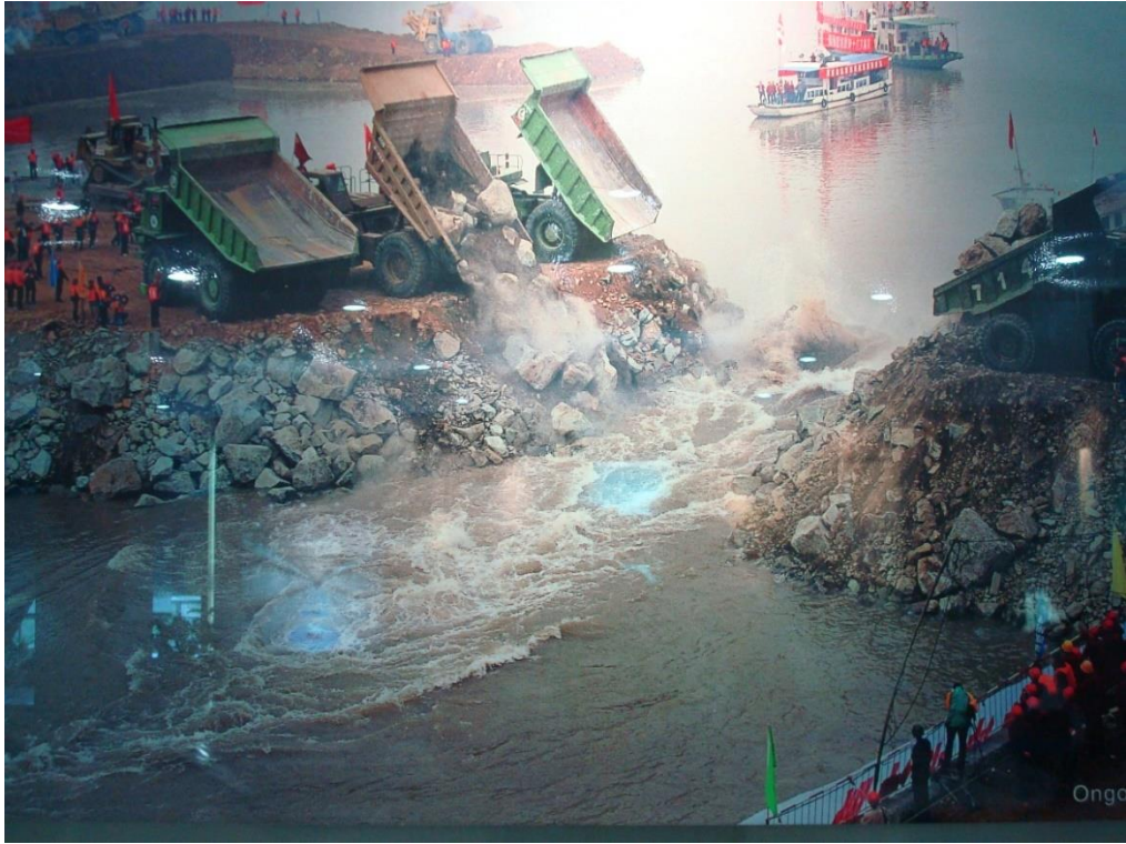
Dumping rockfill material
